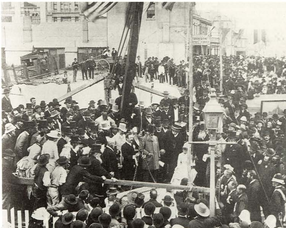
Laying the foundation stone of Trades Hall. Working men in dungarees and flat-brimmed hats clamber onto the platform to get a better view as Lord Carrington declares the foundation stone of the new Trades Hall well and truly laid. Lady Carrington, almost the only woman present, sits between John West (left), president of the Trades and Labour Council, and Sir Henry Parkes. The new hall, on the corner of Dixon and Goulburn streets, Sydney, is located in a shabby neighbourhood of decayed buildings. Carrington departed from the centennial theme to warn against the dangers of slum housing in inner Sydney and to preach the virtues of home ownership: a country gained greater security, he said, where men lived in freehold homes.
